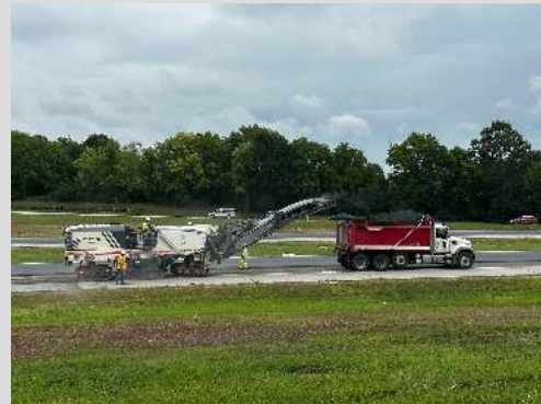
Milling crews working on I-435
