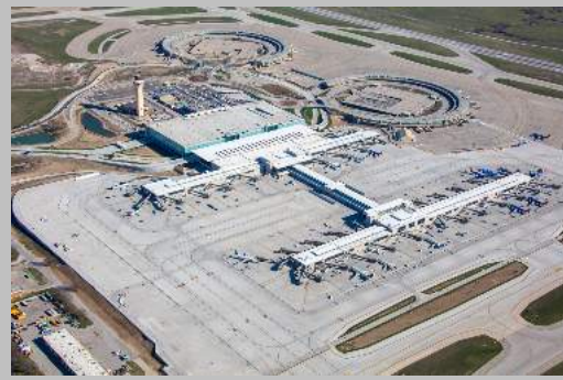
Much of the concrete around the new KCI terminal was placed by Ideker crews
