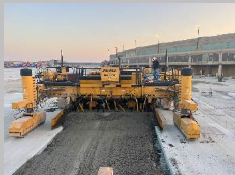
Paving around the terminal at KCI
