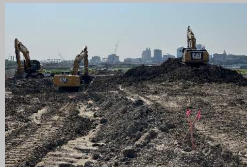
Building the new taxiway at Wheeler airport
