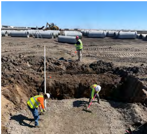
The pipe crew prepares the subgrade for a large manhole box weighing nearly 48,000 pounds.
