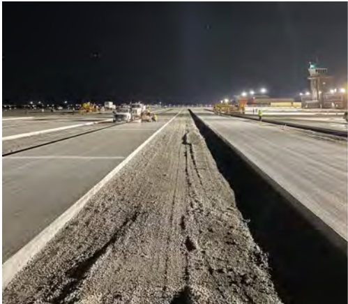
Lights had to be utilized on long days of mainline paving. Paving at night was necessary in order to maximize plant production and to avoid headers.
