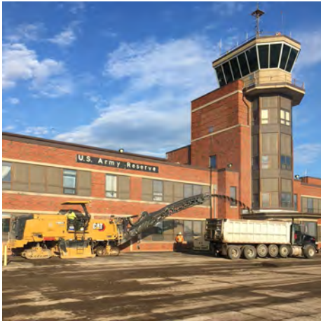
The milling crew removes the old layers of pavement.
