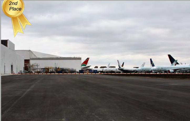
Over 33,000 square yards of asphalt (8,700 tons) was placed to construct the area around the airplane maintenance facility at KCI. The project was awarded the 2nd place MAPA quality paving award for Airports.
