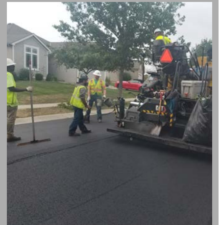
The crew led by Ryan Higginbotham places an asphalt overlay in a neighborhood north of the river near 291 Highway.
