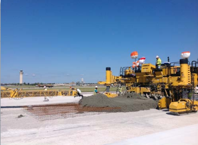
Weather was a huge factor for the concrete paving team, high winds, humidity or air temperature would delay paving for days
