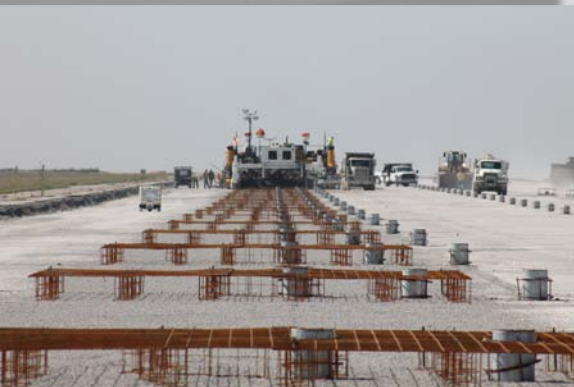
Crews set up and paved around 640 large can lights
